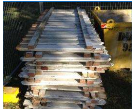
About 8 tonnes of timber picket fencing material had to be disposed of. We were able to achieve reuse of about 80% through selling and giving away the materials.
