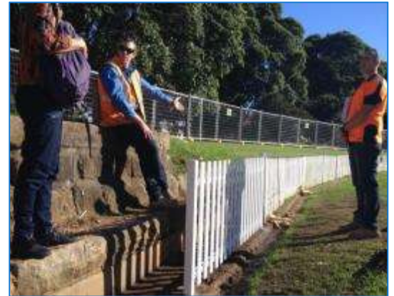
We had various hold and witness points in the project, including the installation of a single panel before proceeding with the works.
