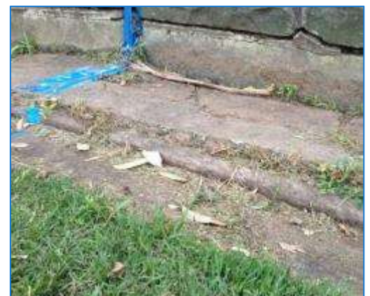
An example of the uneven surface and old fence posts and footings at Petersham Park.
